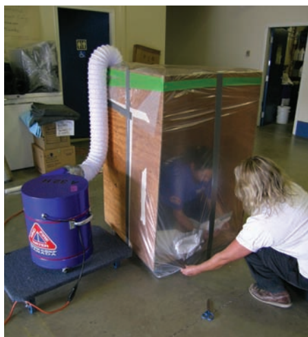
Figure 1a, b, c. Constructing the test chamber and ventilation system. Note the use of existing structures and equipment and readily available materials.
