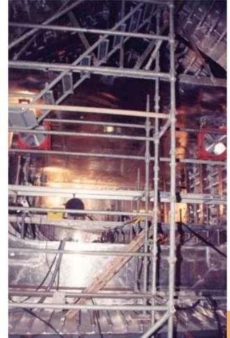
Portable fans were used to ventilate large ship structures during welding.
