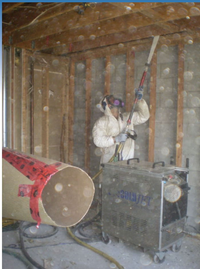
Figure 4 (a, b): Work areas. Dry ice blasting in an open work area (shown following abrasive blasting and application of a sealant) offers greater opportunity for control of exposure than work occurring in enclosed geometries. The latter pose difficult ventilation challenges.
